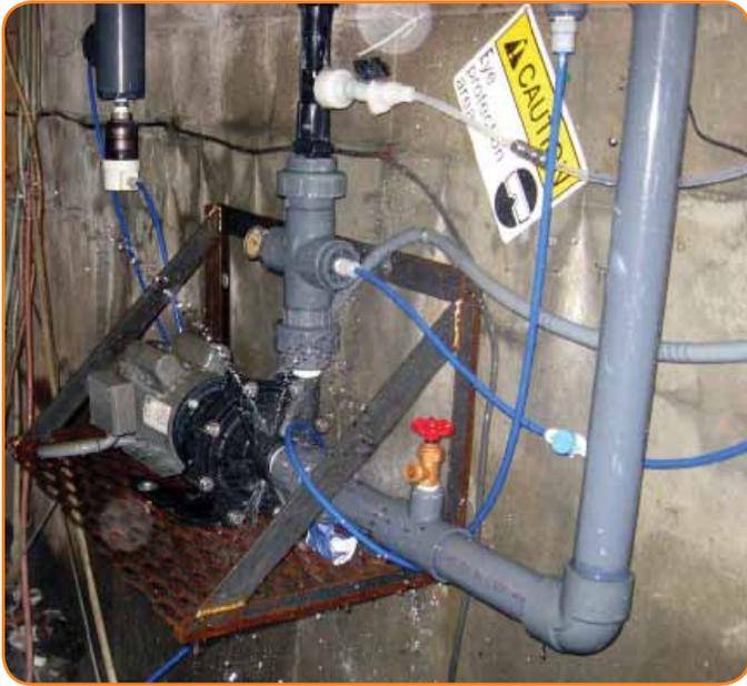
A mag drive pump caused a fluid rupture in a hazardous chemical application, putting workers at great risk.
