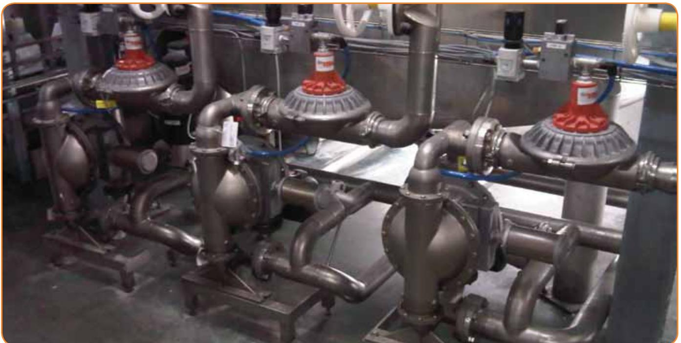
AODD pumps feature strong suction and can provide a "dry prime" by drawing fluid from tanks no matter the location.
