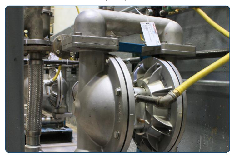
While plastic pumps are typically a go-to pumping technology in chemical processing, there can be instances where metal pumps are a better choice for the operator. Specifically, bolted, ductile-iron AODD pumps from Wilden® can meet the needs of the processor through efficient operation and reliable prevention of leaks and cross-contamination, and they do it at a lower price point than stainless-steel models.
