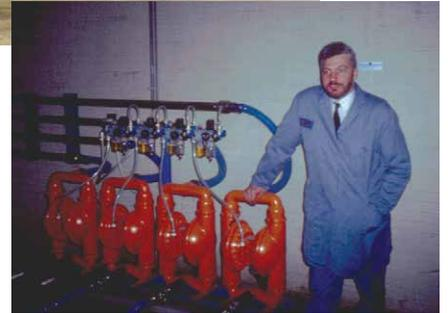
The unique characteristics and requirements of the raw materials that SABA uses and the finalized products it produces also means that stainless-steel pumps with PTFE (Teflon®) diaphragms, elastomers and check balls are required. Wilden delivers that to SABA with its Original™ Series PX4 and PX8 (1.5 and 2 inches; 38 and 51 millimeters) clamped AODD pumps and Advanced™ Series PX400 and PX800 bolted AODD pumps.
