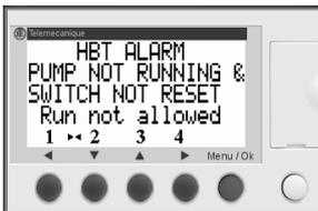
Indicates that the liquid in the Storage Tank has exceeded the maximum allowable temperature while the Pumpset is NOT running, tripping the HBT switch. The Pump Controller will not allow the Pumpset to start until the HBT switch automatically returns to its normally closed position.
