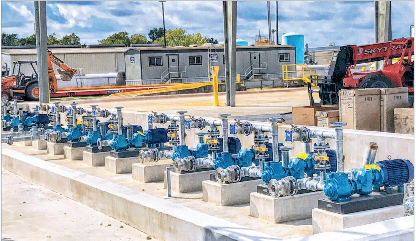
While many chemical fluid-transfer operations may take place in harsh environmental conditions, the pumps and systems used to facilitate product transfer are in actuality delicate ecosystems that must be kept in balance and operate in harmony. Therefore, any upset in the system - including improper shaft alignment - can result in breakdowns that can lead to excessive downtime and high repair or replacement costs.
