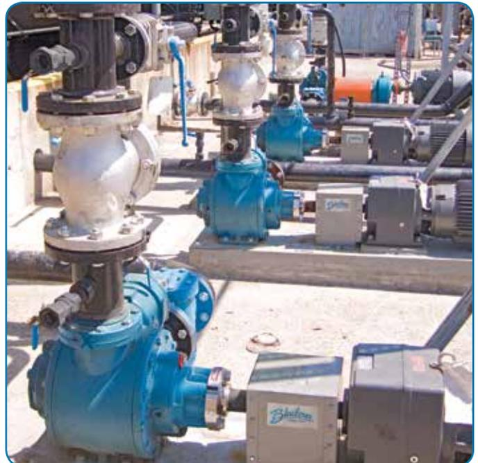
**Blackmer® Smart Energy® Sliding Vane Pumps can be a critical energy-conscious component in a soap and detergents manufacturing operation.**
