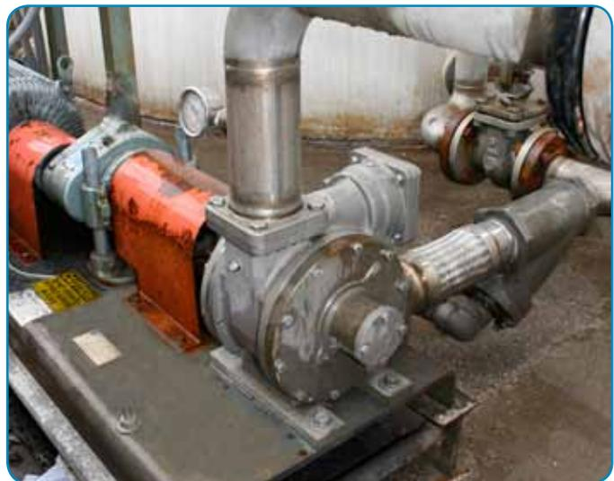
Blackmer SNP Series Sliding Vane Pumps (pictured) are ideal for use in various feedstock transfer applications found in and around soap and detergents manufacturing plants.
