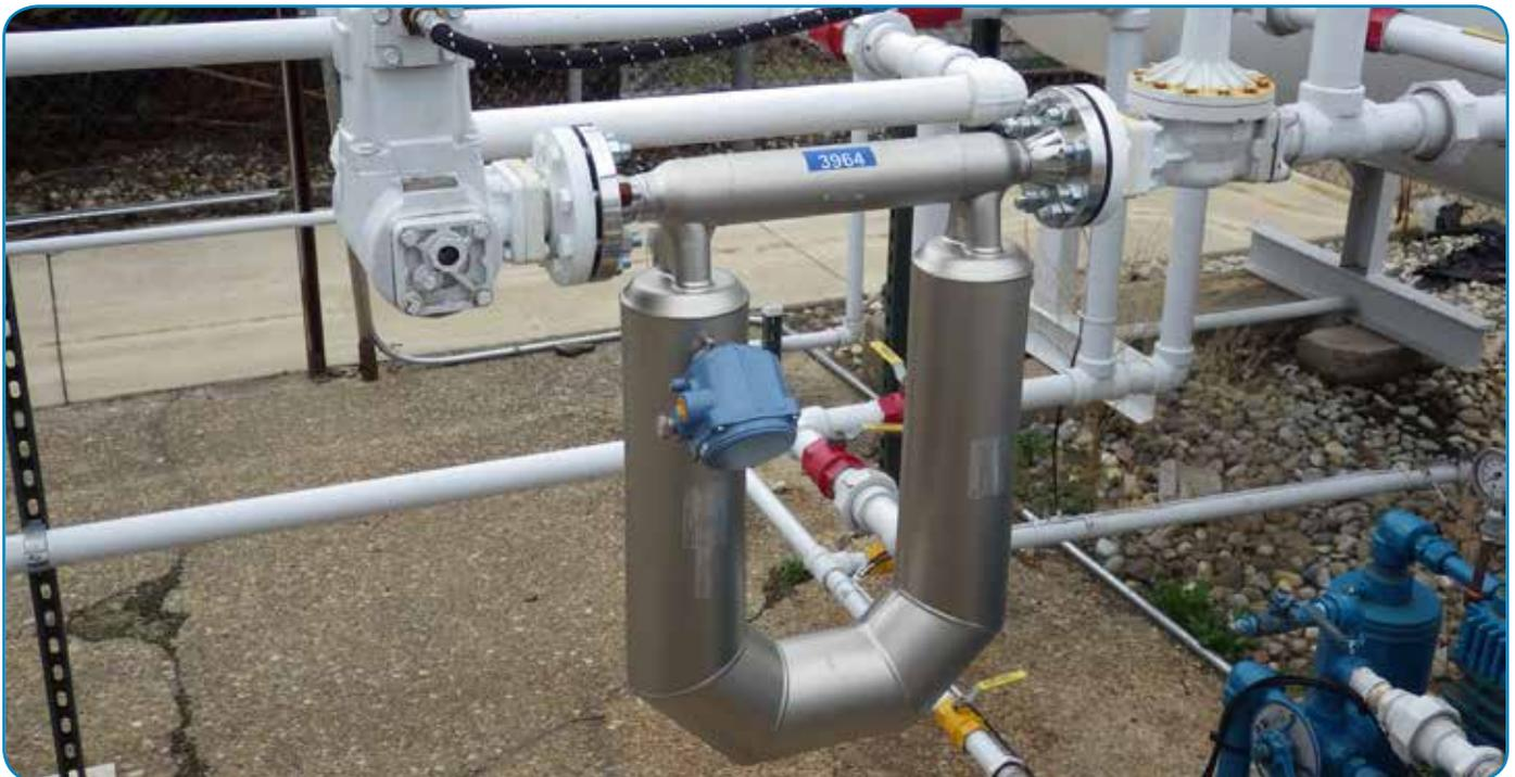
Figure 1: Emerson Mass Flow Meter Installed horizontally on Propane (LPG) System
