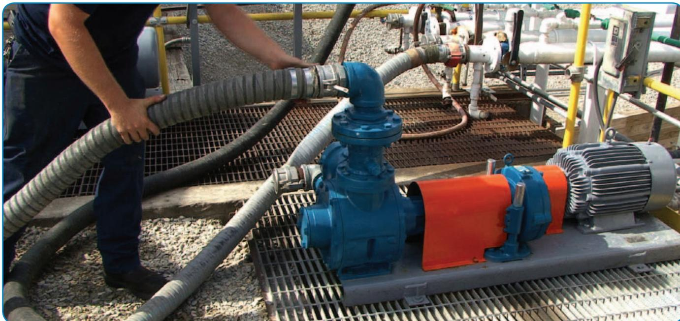
Demands put on liquid-storage terminals appear to be at cross-purposes: maximize throughput while minimizing energy consumption. Nevertheless, sliding vane pumps provide a transfer technology that offer streamlined, reliable operation while consuming low amounts of energy.
