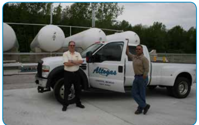
Jim Becker, left, and Scott Tonkin, in front of the facility's four 30,000-gallon LPG storage tanks.
